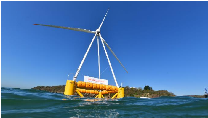
A prototype floating wind turbine in the test phase © Ifremer-Eolink - O. Dugornay
